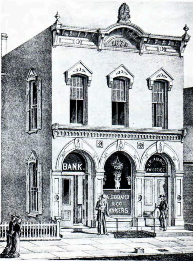
THE FIRST NATIONAL BANK building, erected in 1875, is now the Conway Photo Stop. The bank moved to a new building at Church and Grove streets in 1953 and is now the National Bank of Northern New York.
