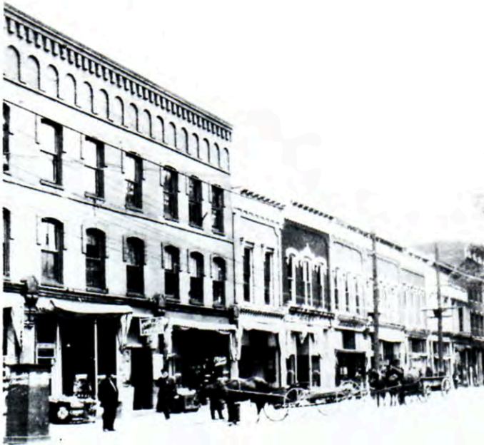
View of the new brick buildings constructed after the 1877 fire toward the Clinton Street end of Main Street.
