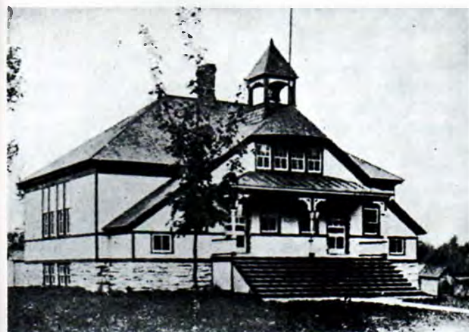
THE SOUTH SIDE SCHOOL opened in 1890 on Depot Street and burned in 1934. It was not replaced.
