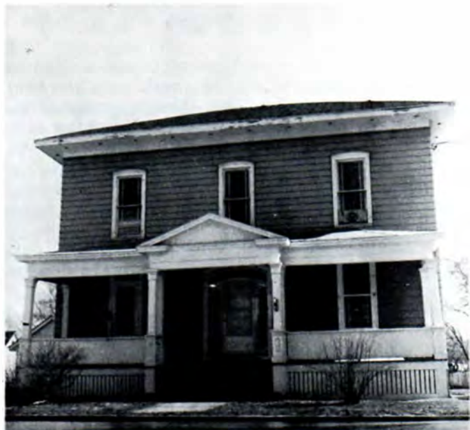
HOME OF BENJAMIN HOWARD SMITH (120 E. Barney St.). This house was moved from its original site on the corner of Barney and Rock Island Streets to make way for the Dean High School.
