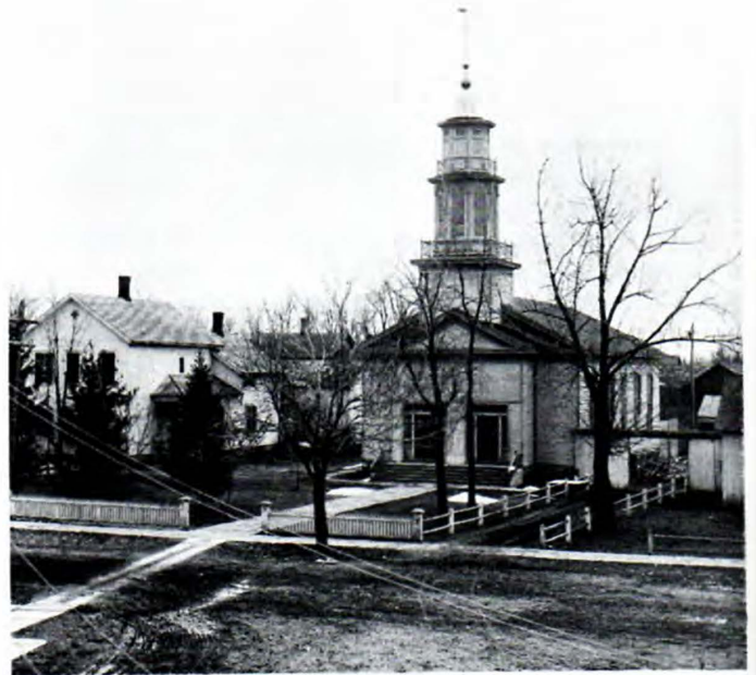
PRESBYTERIAN CHURCH AND MANSE — The second building built in 1844 by the Presbyterian church replaced a small, rough building started in 1820 and completed in 1824. The house to the left of the church was the manse. The Presbyterian churches have all been on the same site.
