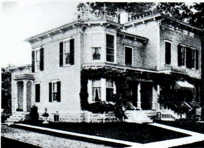
DR. CARPENTER'S HOME at 29 Grove Street.
