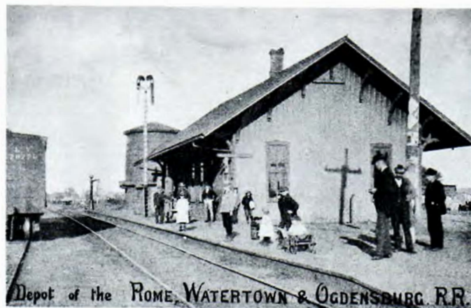
OLD RAILROAD STATION
