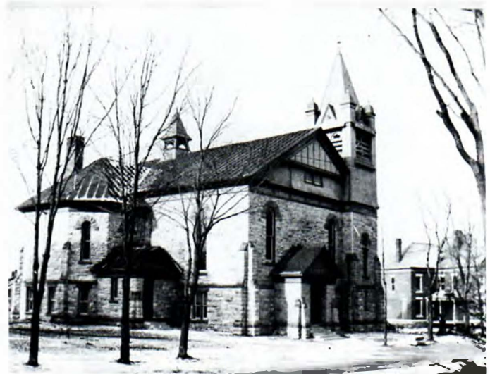
THE METHODIST CHURCH built of sand stone in 1871, was remodeled and faced with marble in 1891.
