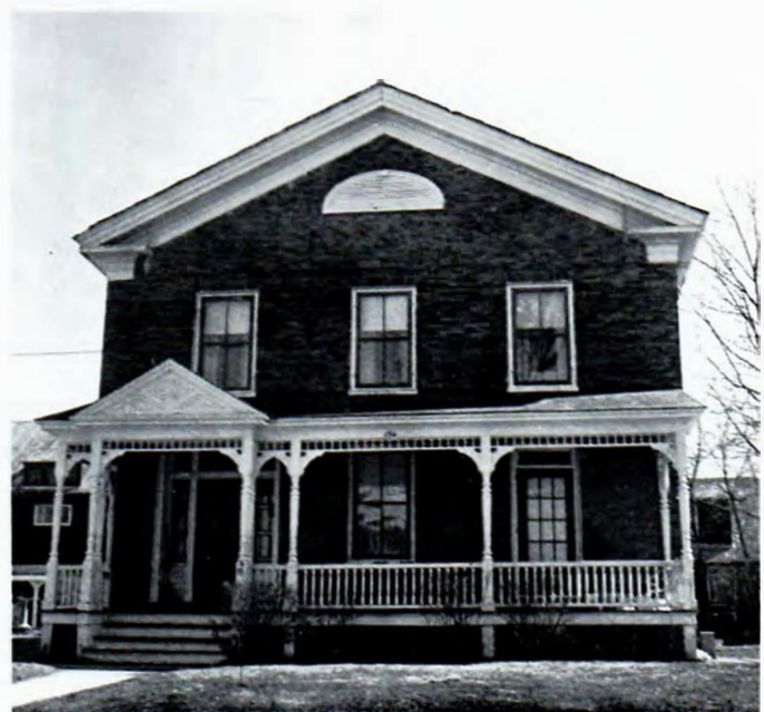
The William E. Sterling house , 174 East Main Street
